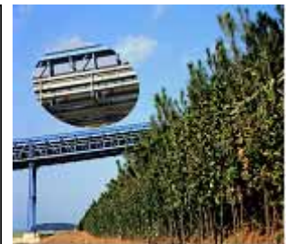
[炭塵飛散防止設備]
